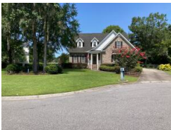
4203 Links Court North Charleston SC
